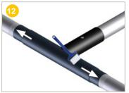
While the sleeve surface is still hot and malleable, use the application roller to **smooth** and **evacuate** the air bubbles.
