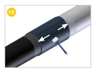
While the sleeve surface is still hot and malleable, use the application roller to smooth and evacuate the air bubbles.
