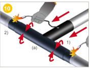
1) **Slide** the large heat-shrinkable sleeve (a) around the HDPE muff (b).
