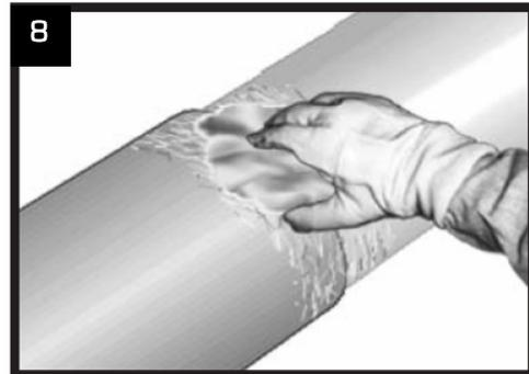
Clean the corrugated surface to remove any particle of polyethylene or sand by using a dry rag or the breath of the flame.
