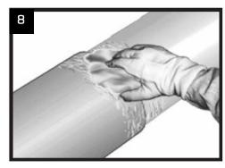
Clean the corrugated surface to remove any particle of polyethylene or sand by using a dry rag or the breath of the flame.
