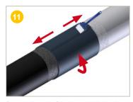
**Press** both ends of the heat-shrinkable sleeve firmly.
